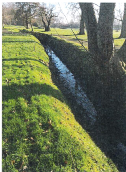
Photo 3: Well maintained, free-flowing ditches were seen throughout
